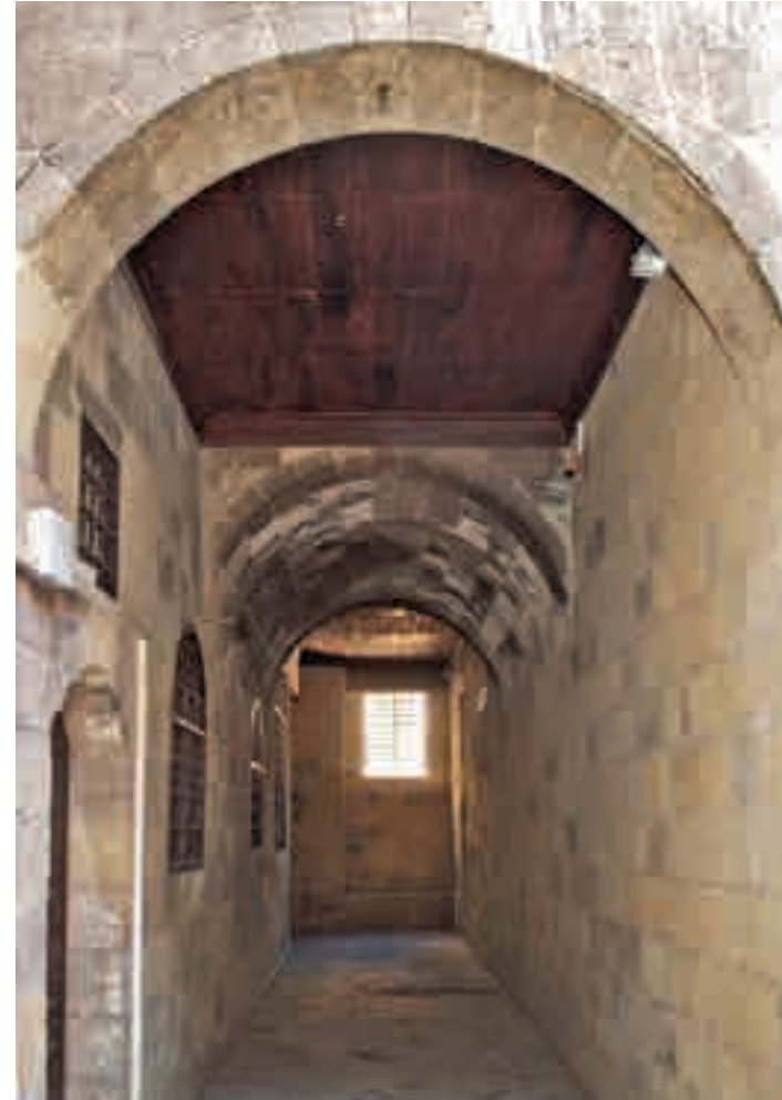
(Picture 18) The entrance corridor from the internal yard towards the outside
