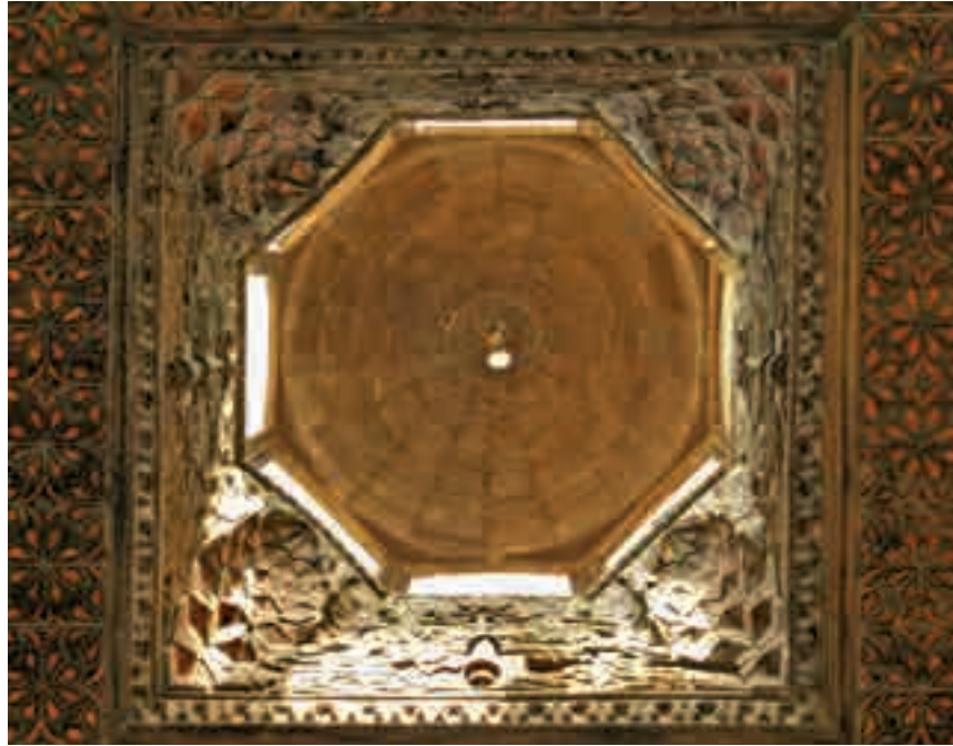
(Picture 72) The grand hall, the derkah, the octagonal shoukhsheikha that is in the middle of the wooden ceiling of the derkah. It is based on skillfully made wooden stalactites
