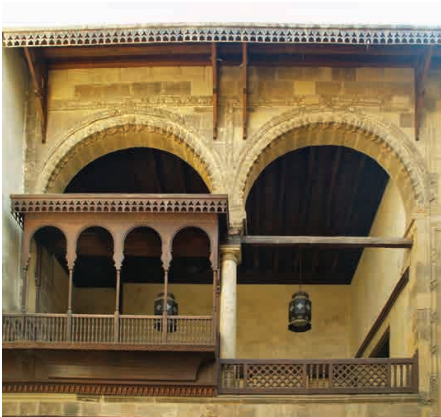
(Picture 29) The seat façade
