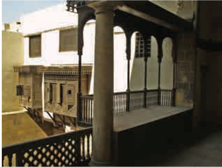
(Picture 49) Reception areas, the seat from the inside, the protruding wooden roushen overlooking the main yard
