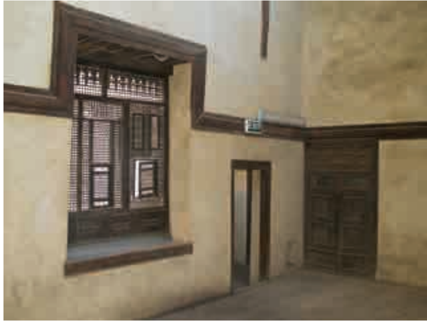
(Picture 67) The area in front of the grand hall, the entrance to the grand hall and the window covered with a screen of etched wood overlooking the derkah of the grand hall
