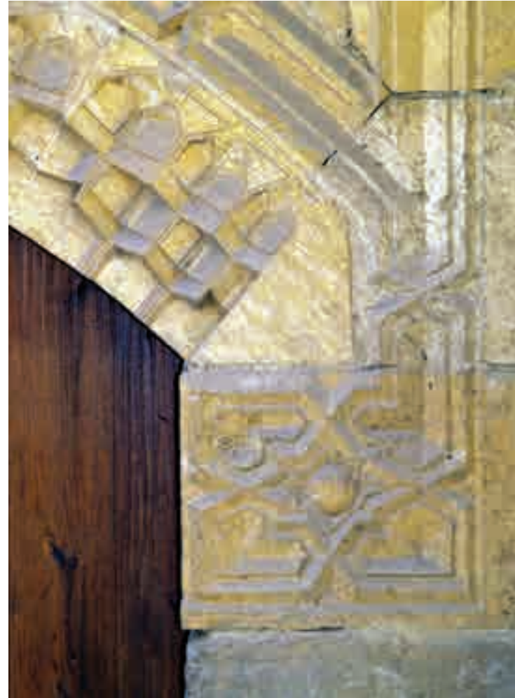
(Picture 13) The entrance block, details
