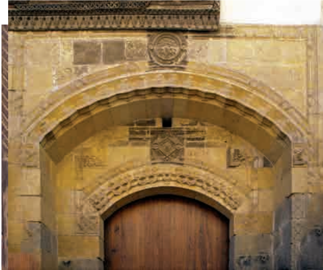
(Picture 11) Tendoned arches crowning the main entrance opening
