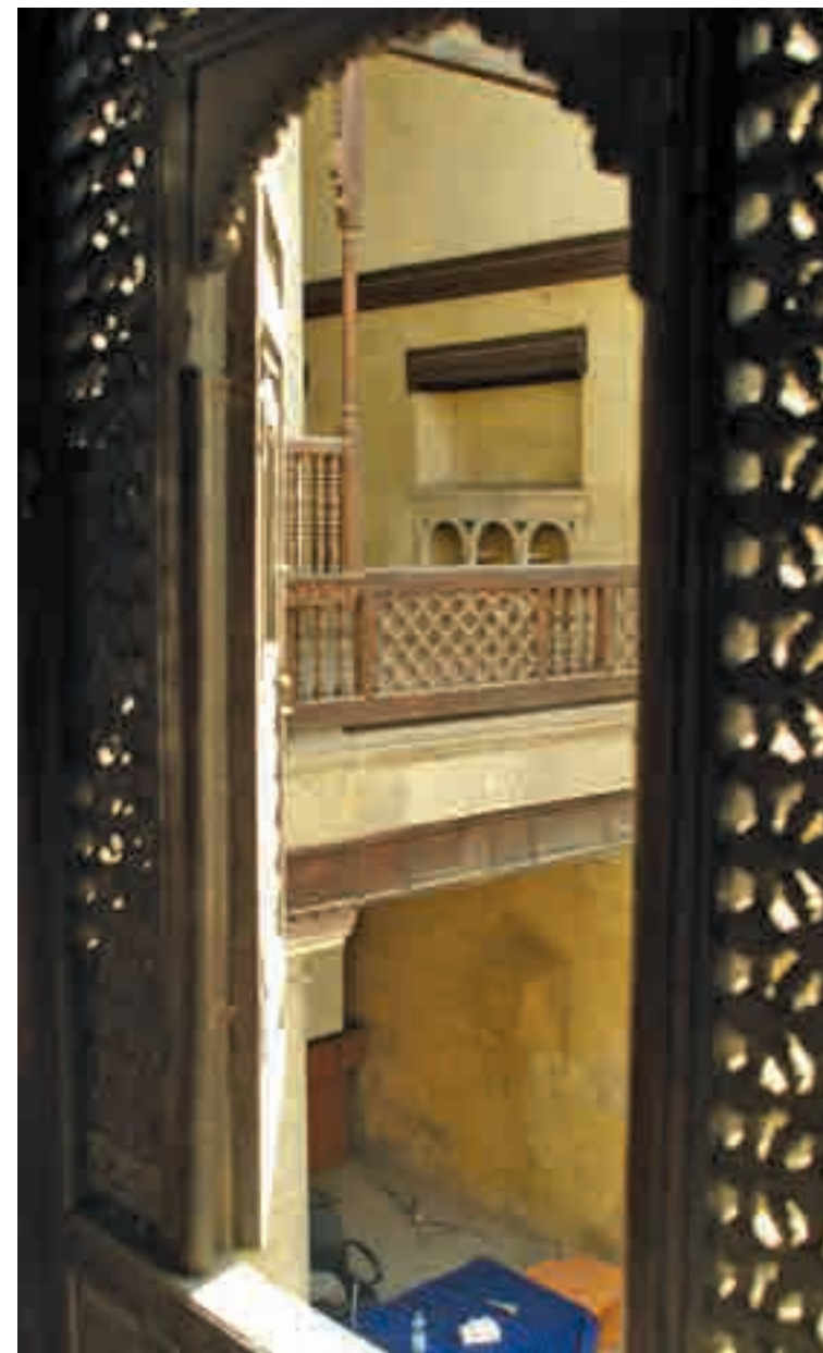
(Picture 60) Reception areas, the Harem hall, from inside the sudla of the south western iwan and its Mashrabeya overlooking the yard, the seat and the takhtaboush
