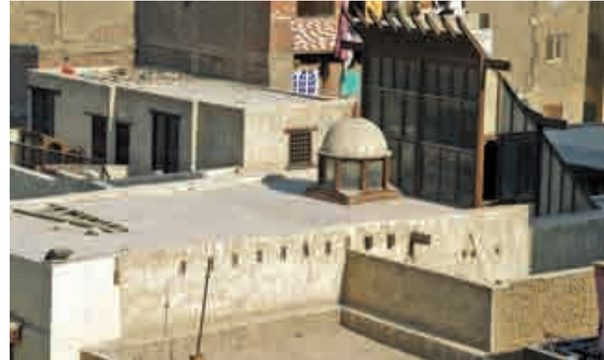
(Picture 89) The ceiling of the house. The large ventilation skylight and the dome to air the grand hall can be seen. To the left of the picture is the small wooden ventilation skylight used to air the rooms and areas in the Harem section
