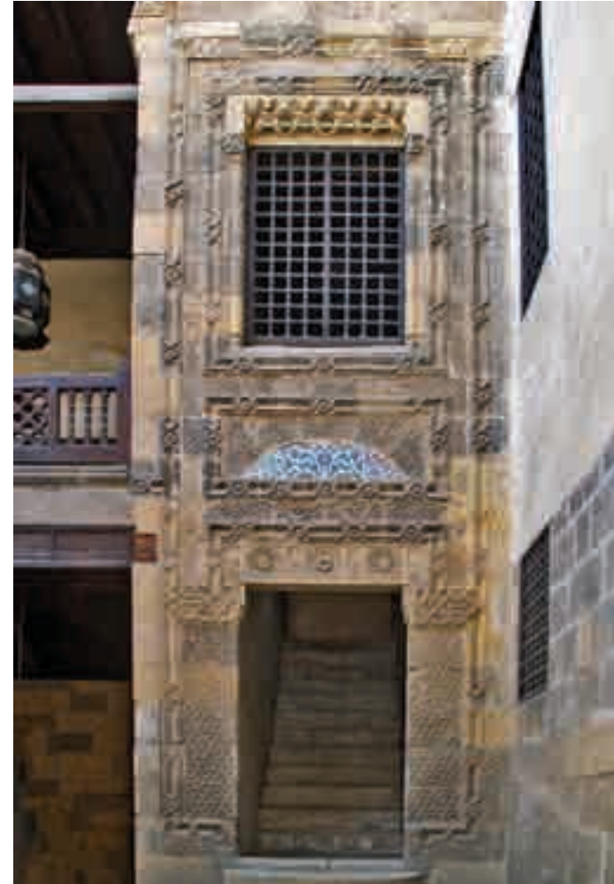
(Picture 25) The seat entrance block
