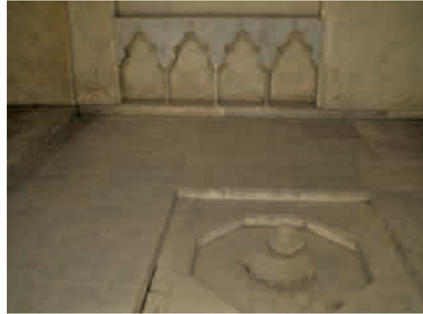
(Picture 73) The grand hall, the derkah, the fountain in the middle of the derkah, with a mural niche in the middle of the inner wall, below which is a marble arcade of four arches used to place lamps and the various needs of the hall
