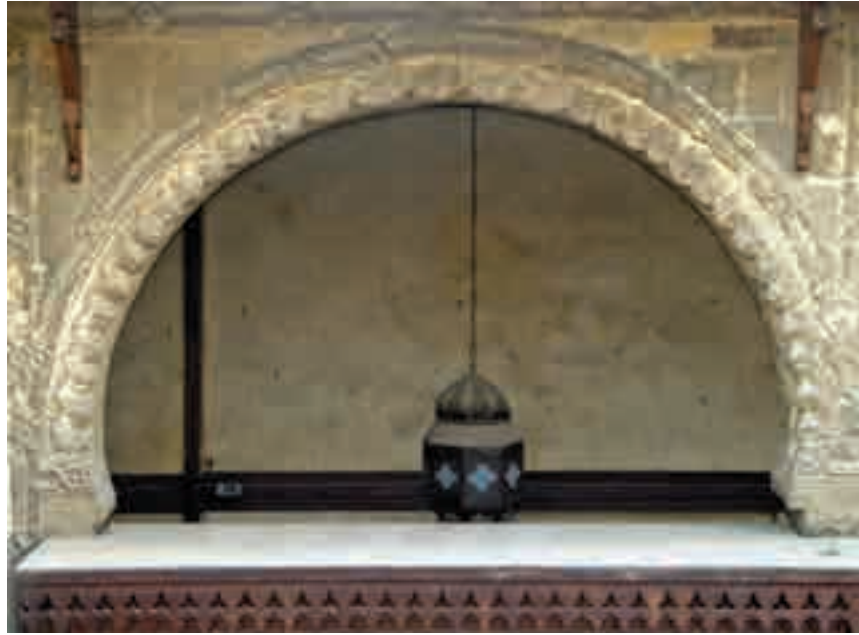
(Picture 30) Details of the seat façade arch
