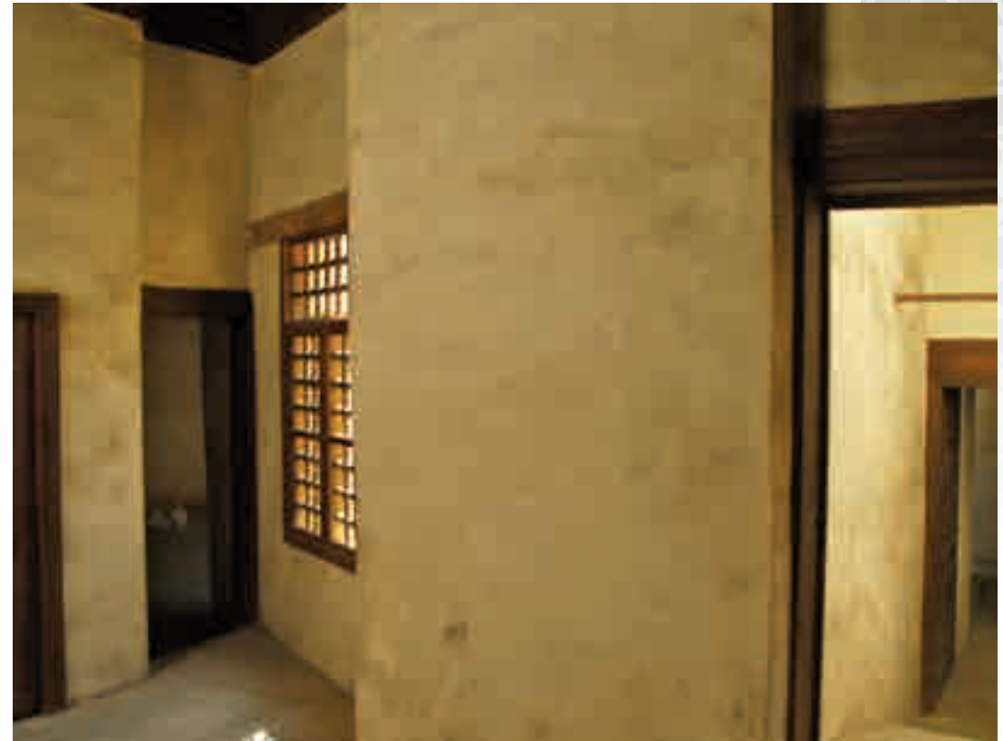
(Picture 81) The area around which the Harem rooms are distributed on the first floor. To the right of the picture, there is door to the secondary yard stairs. To the left of the picture, there can be seen the slope in the secondary yard wall on this side, intended to make space for the door to one of the rooms
