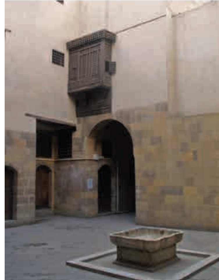
(Picture 19) The main yard, the arched corridor opening that leads into the yard, above it a Mashrabeya
