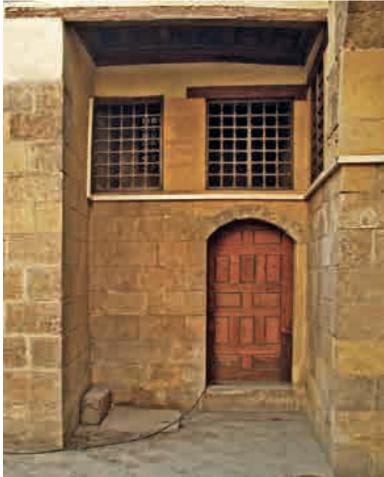
(Picture 22): The main yard, the western corner is a recess in front of the service areas
