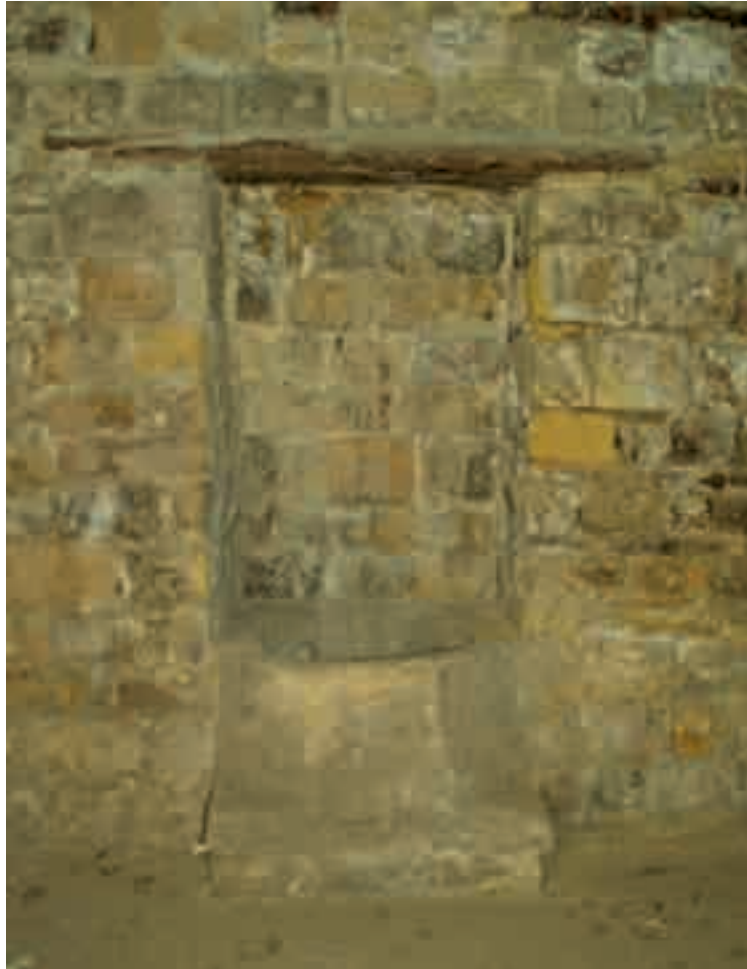
(Picture 36) A water basin in one of the services areas that opens onto the secondary yard
