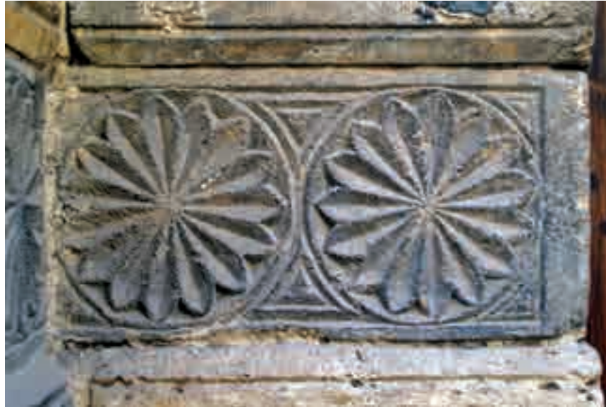
(Picture 14) The entrance block, motifs etched in stone
