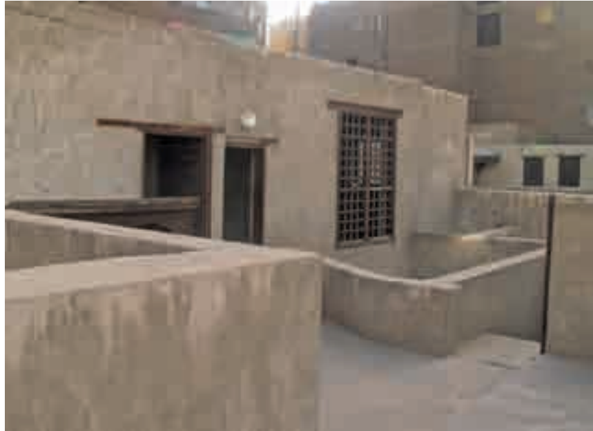
(Picture 84) The area on the second floor in the Harem section, onto which two rooms open. There is the ventilation skylight which receives the air for the area beneath it on the first floor
