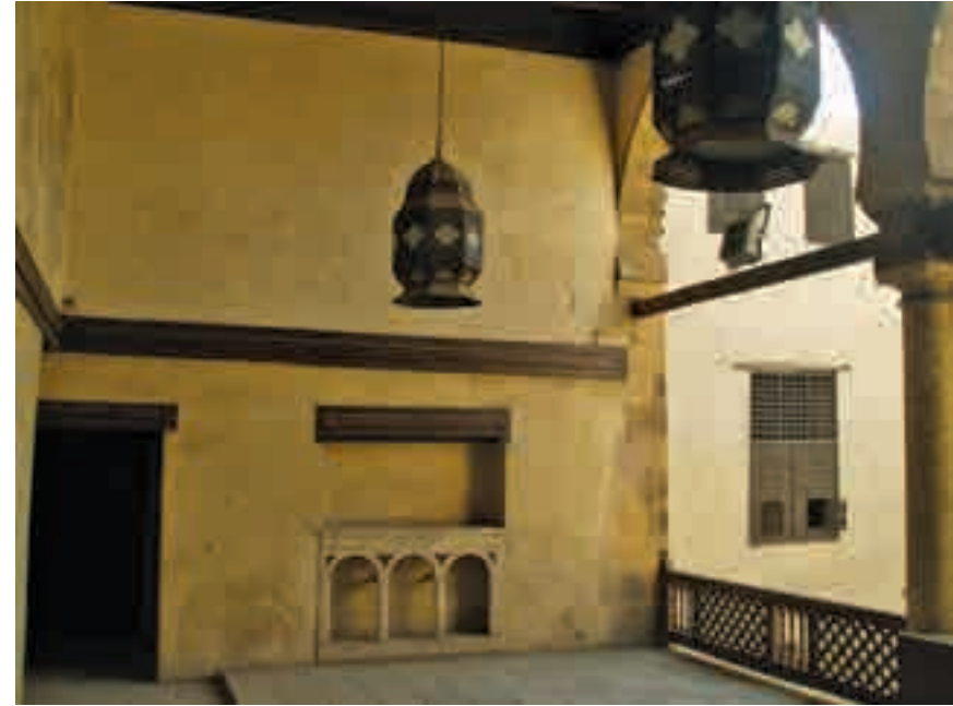
(Picture 46 ) Reception areas, the seat from the inside, the western section, at the center of the wall of which is a niche with marble
