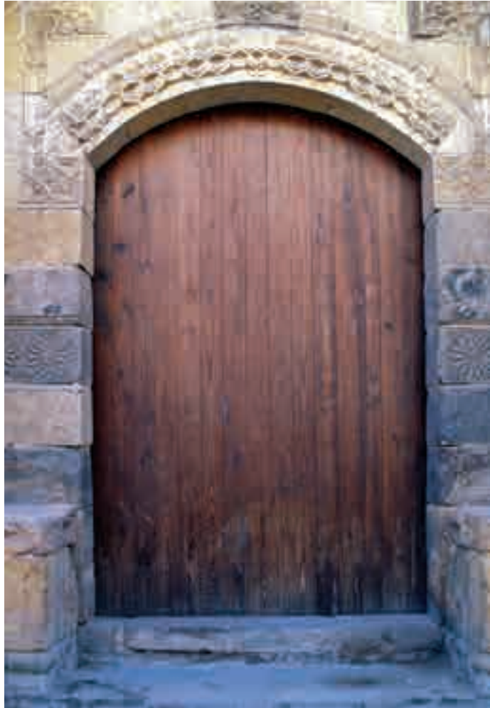
(Picture 12) The entrance block, main entrance opening
