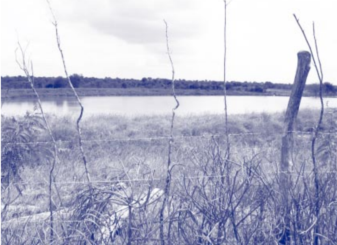
Katutuni Community Earth Dam provides clean water for 3000 residents of Makutano.
