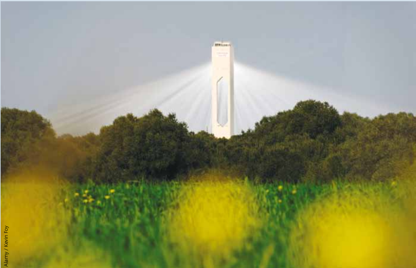
The solar tower in Andalusia, Spain. Six hundred mirrors reflect sunlight to produce steam for electricity generation.
