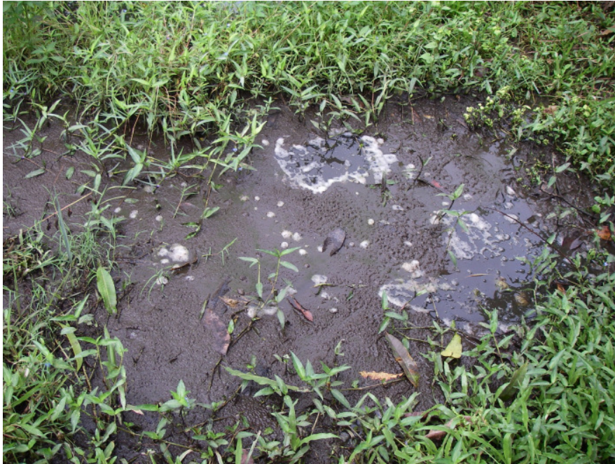
Image: A poorly built and maintained slurry pit with no lining and no protection from rainwater infiltration. Slurry from this pit had lower levels of nutrients, probably due to dilution with rainwater. Inconsistent nutrient levels and the small size of digesters make slurry less attractive for commercial producers of fertilizer and compost.
