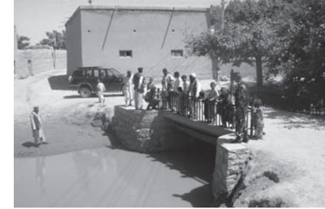
A new small bridge in Aliabad, Northern Afghanistan.
