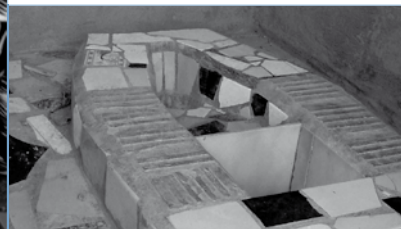
Ownership fosters creativity, as seen here by the example of this nice self-made urine-diverting squatting seat in Kyrgyzstan
