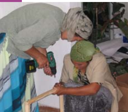
Women in Kyrgyzstan are building a solar warm water heater Picture source: WECF partner BIOM, Kyrgyzstan
