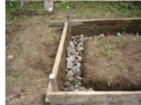
Figure 46: Foundation is being prepared
