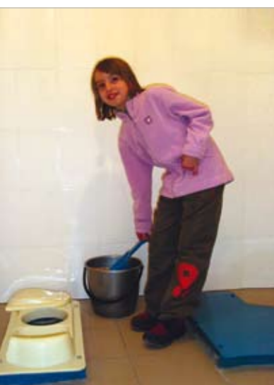
Figure 25: One of the 4 new urine diverting toilets of the school. The toilet on the left will be used until the faeces chamber is full, after which it will be closed for two years to give the collected faeces time to sanitise
