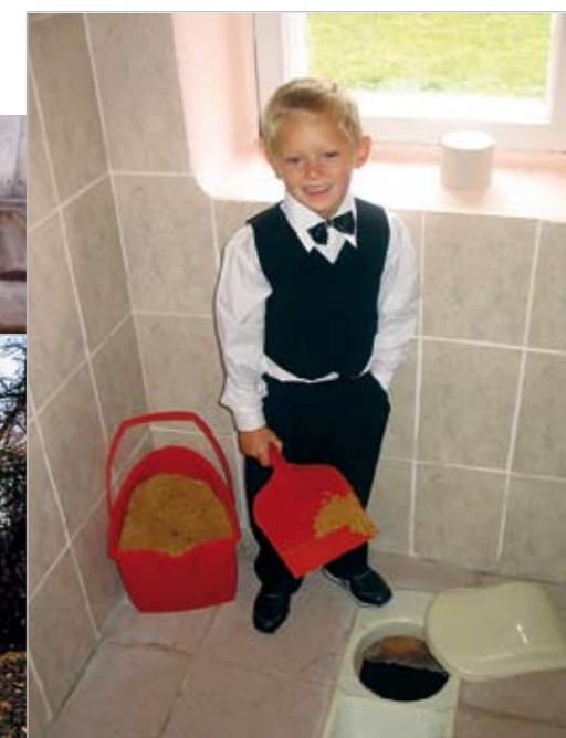
Figure 12: This toilet is one of the first examples of an indoor ecosan school toilet in Ukraine, has no bad smell and is hygienic. The boy shows how one should cover the excrement with soil or wood chips after a toilet visit
