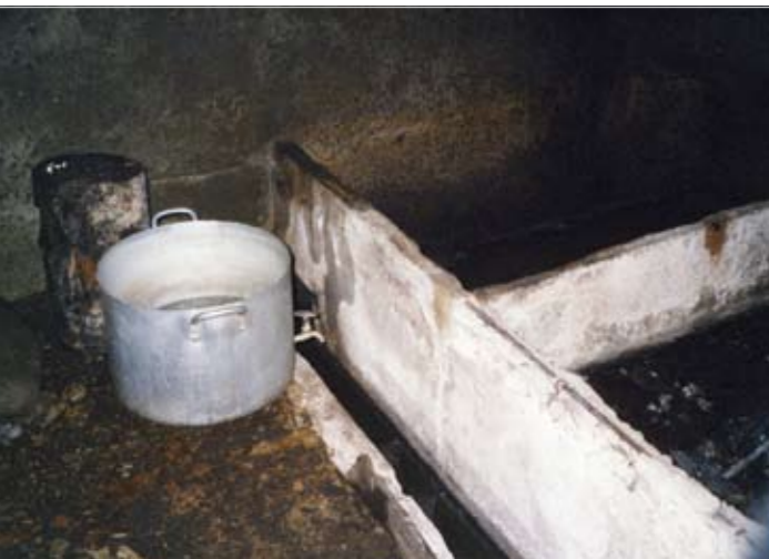
Figure 42: The drinking water treatment of the old central supply system of Vorokhta consists of a pan that is slowly adding hypochlorite to the water
