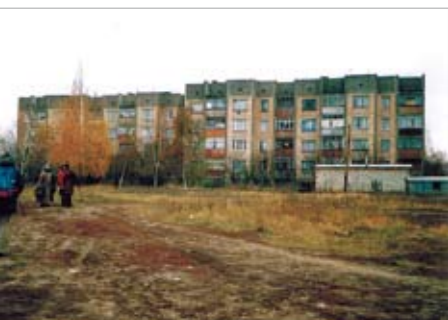
Figure 16: These apartments in Gozhuly were built in Soviet times by factories and kolkhozes for their workers, but since their bankruptcy services, like the maintenance of the central water supply and heating system, discontinued
