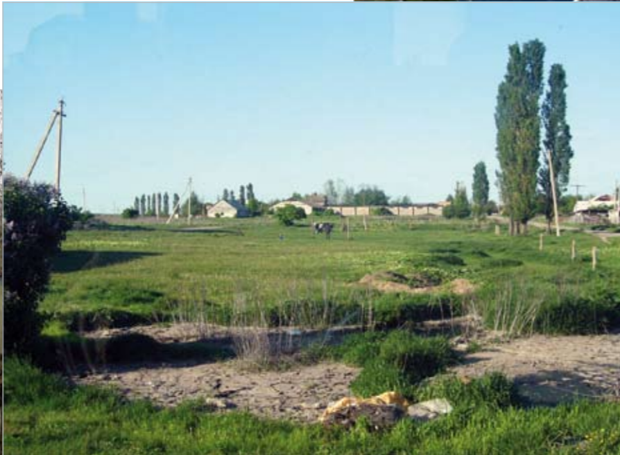
Figure 18: Sewage pipes are rotten, so waste water is on the streets and even in the water catchment area
