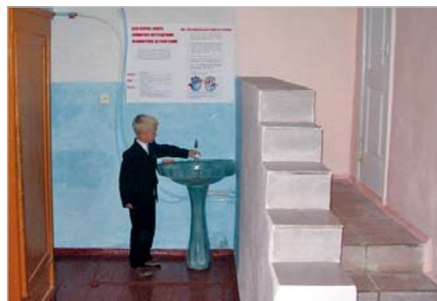
Figure 9: The project team constructed an indoor water connection for hand washing, accompanied by an educational poster explaining why and how to hand wash
