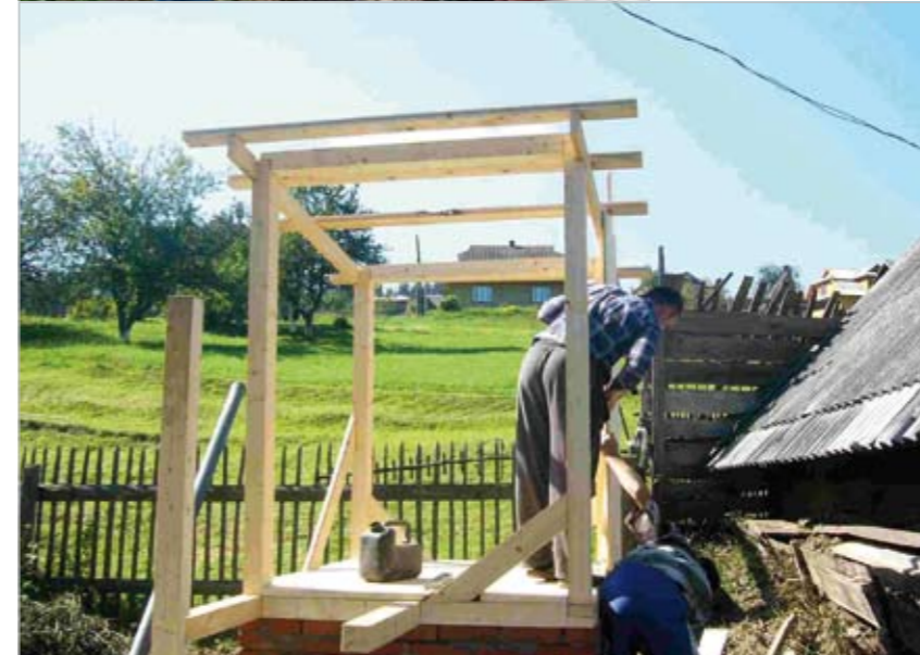
Figure 47 - 48: The frame of the ecosan toilet is being constructed
