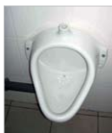
Figure 29: All but one flow-off holes were blocked in each urinal to minimise the interaction between urine and air
