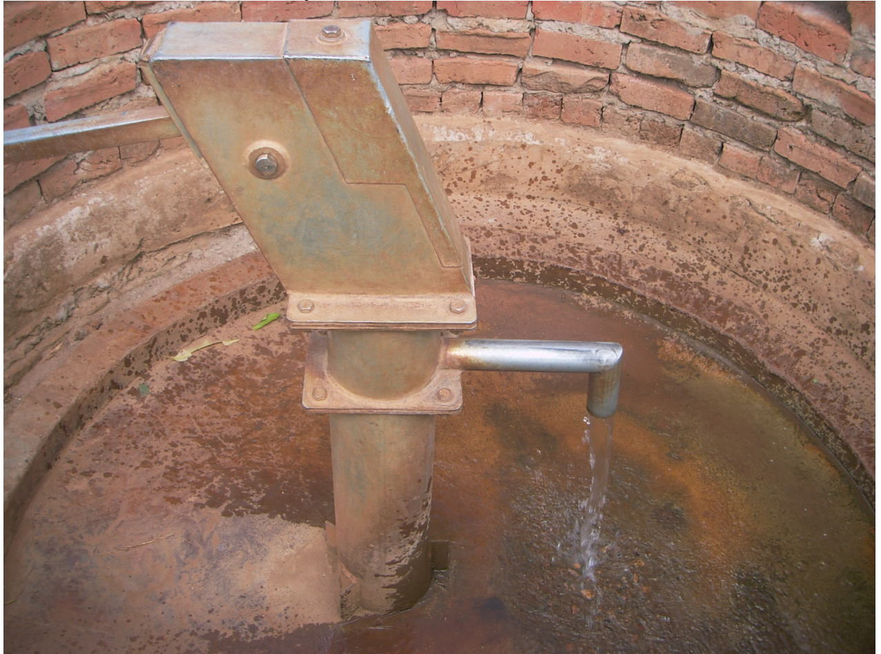
One of the boreholes constructed by GCPDO in Mndemba area
