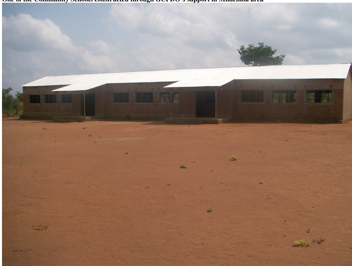
One of the Community Schools constructed through GCPDO's support in Mndemba area
