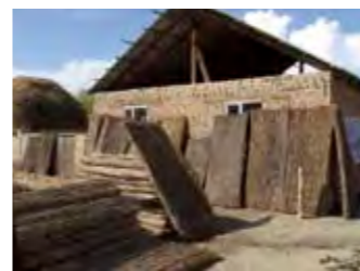
The first straw bale building in the region is being constructed
