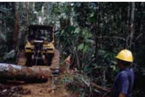
Photo 10.3. The tracked skidder shown here is a D4, so it is relatively light and damages the soil under the skid road but little. It is however strong enough as a mobile winching station, which is its main use. (Photo N.R. De Graaf)
