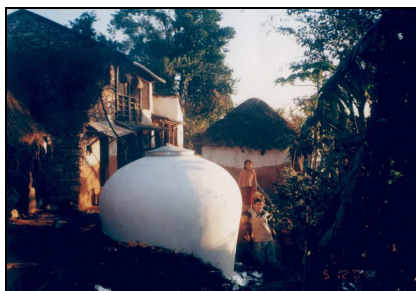
Pictures from left to right: (i) 6,500 litre ferrocement tank shining in the morning sun in Ghaderi Khairikot, Nepal. (ii) Proud owners of a 10,000 litre ferrocement tank in Ouahigouya, Burkina Faso. (iii) Waiting in line to get rainwater from a 40.000 litre tank in Hantezo Bubisa, Ethiopia (© RAIN)
