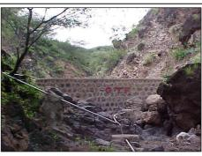
Right: <u>Sand dam water harvesting</u> in Ethiopia (sand and water accumulate upstream from a small dam in a river; water is extracted from the sand)
