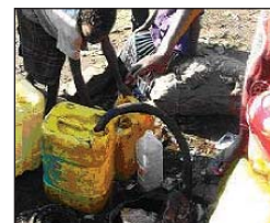
One of the public taps whose pipes have been removed and a garden hose attached.
