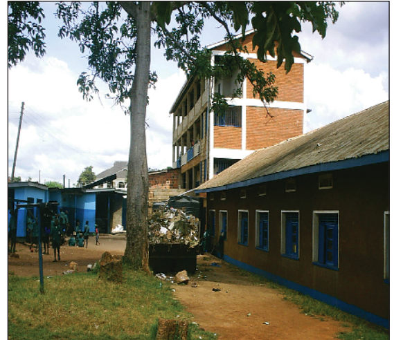
A garbage skip next to the classrooms, Kibuli, Kampala, Uganda.
