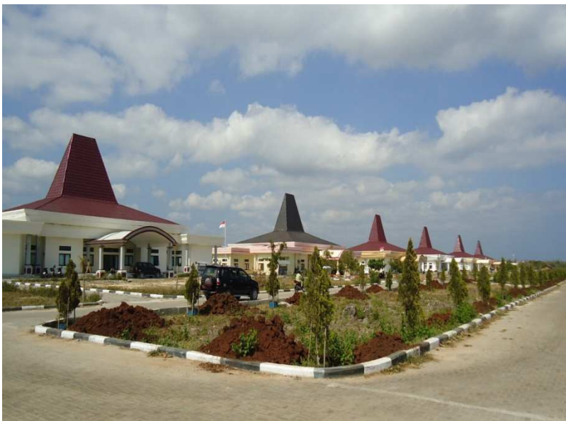
Figure 4. New Sumba Barat Daya government offices
