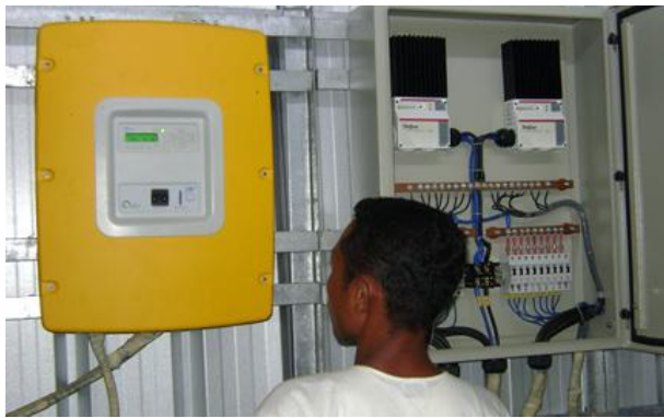
Figure 44: 5 kW Photo voltaic system and solar PV pump system
