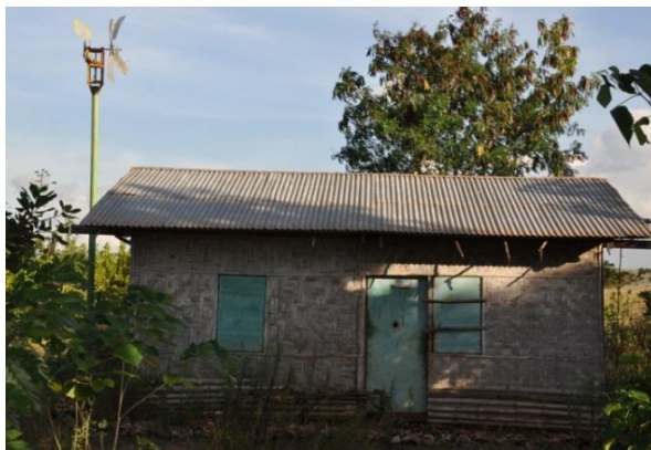
Figure 3: 10W Stand alone wind turbine and PV for communication applications
