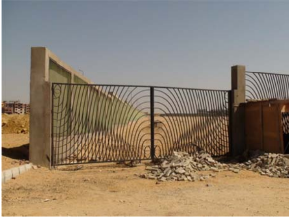
13 Site gate at the northeast
