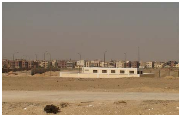
06 Electrical plant facing the site
