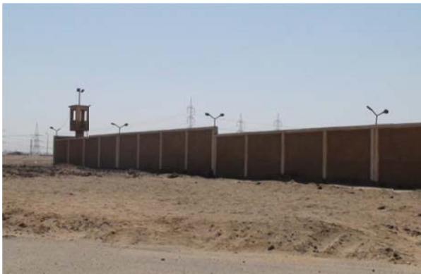
05 Electrical plant area
