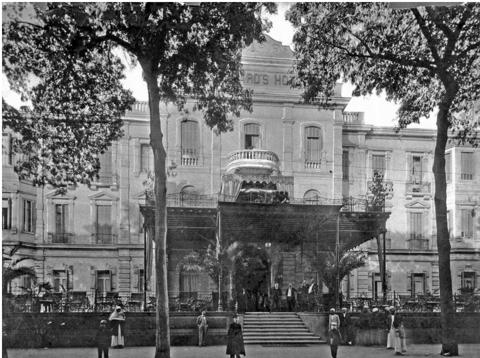
Shepherd Hotel building after reconstruction in Cairo.
