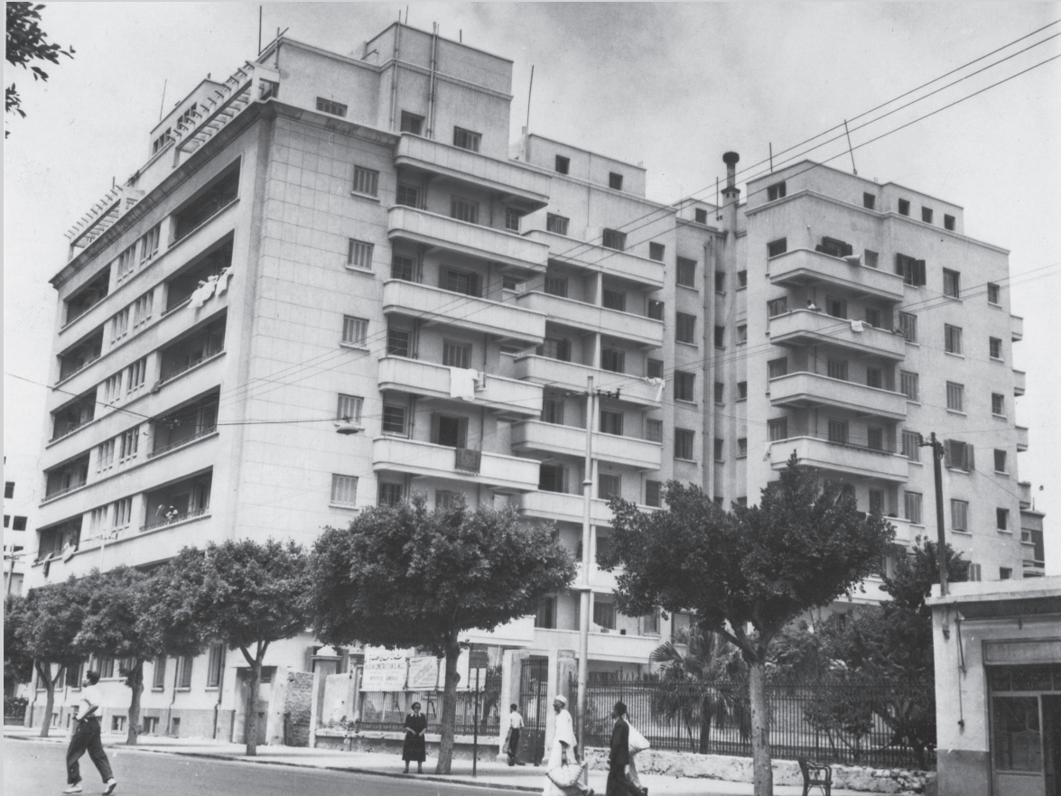
The Heikal H Building: the balcony goes all the way around to the other south side.
