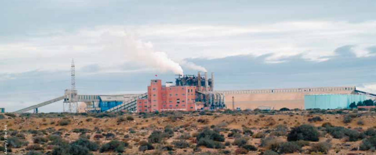
A phosphate factory in Western Sahara, Morocco.
