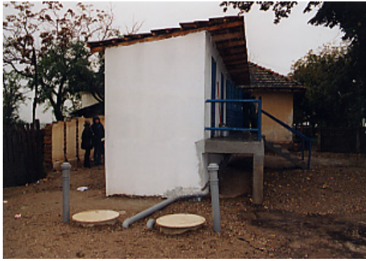
Fig. 6 Front: Urine reservoirs buried under the soil (Source WECF).
