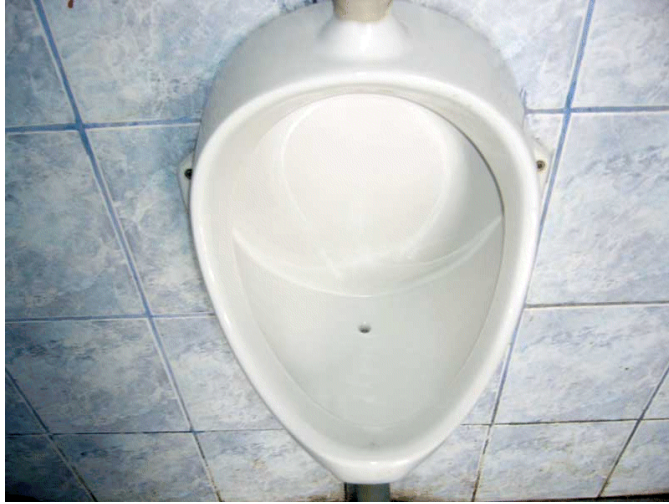
Fig. 12 Improved waterless urinal with one small hole; the other holes have been closed (Source S. Deegener, TUHH)
