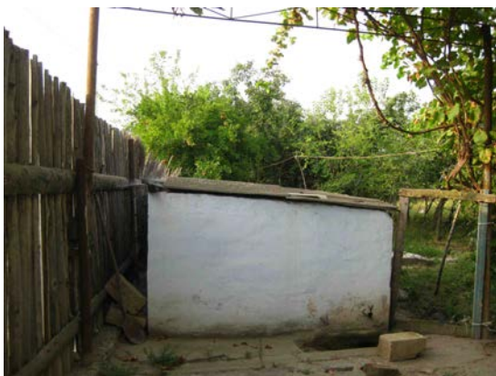
Photo: Basin for the storages of river water
